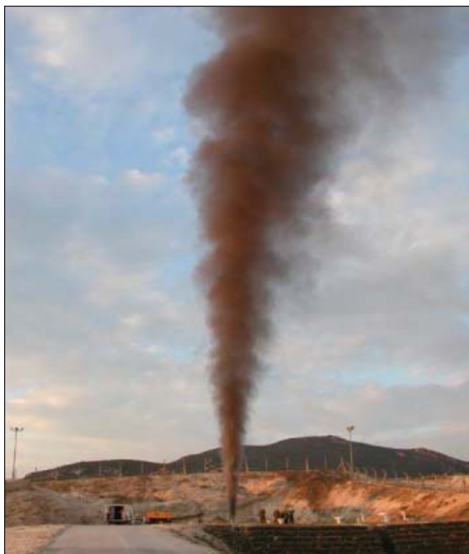
DEPA purged the valve station at the entrance of the border metering station with gas after pigging in order to dispose of any remaining powder and prevent rapid clogging of the cartridge filters, venting large amounts of black powder in the process (Fig. 5).
